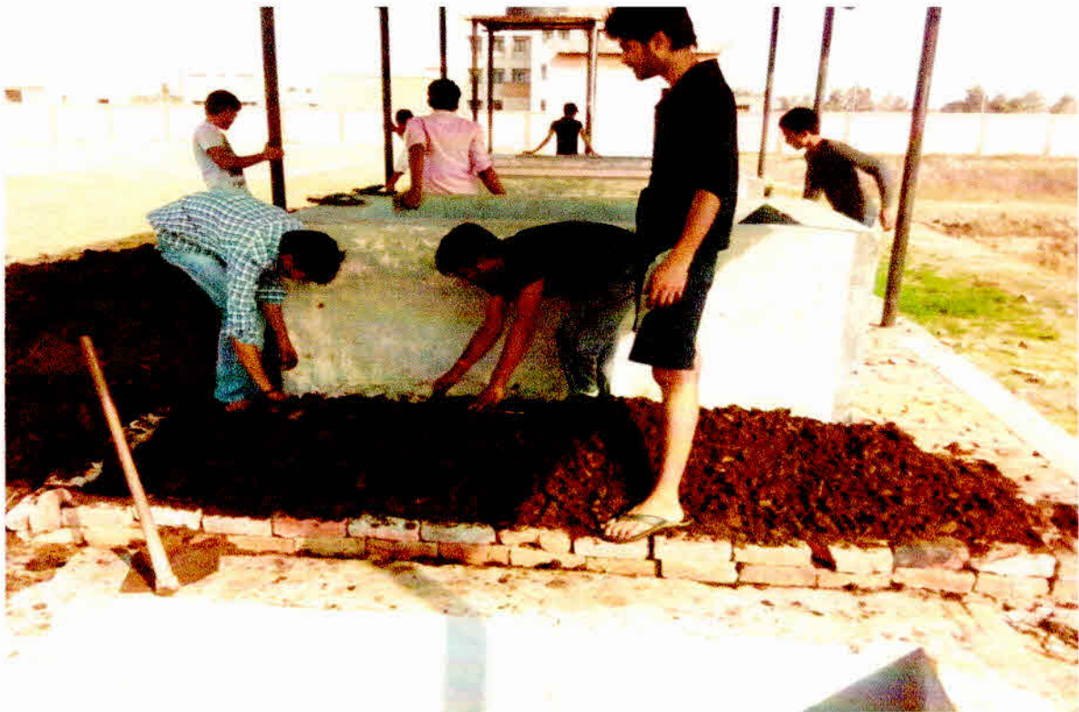
Preparation of Bed in Vermi compost unit
